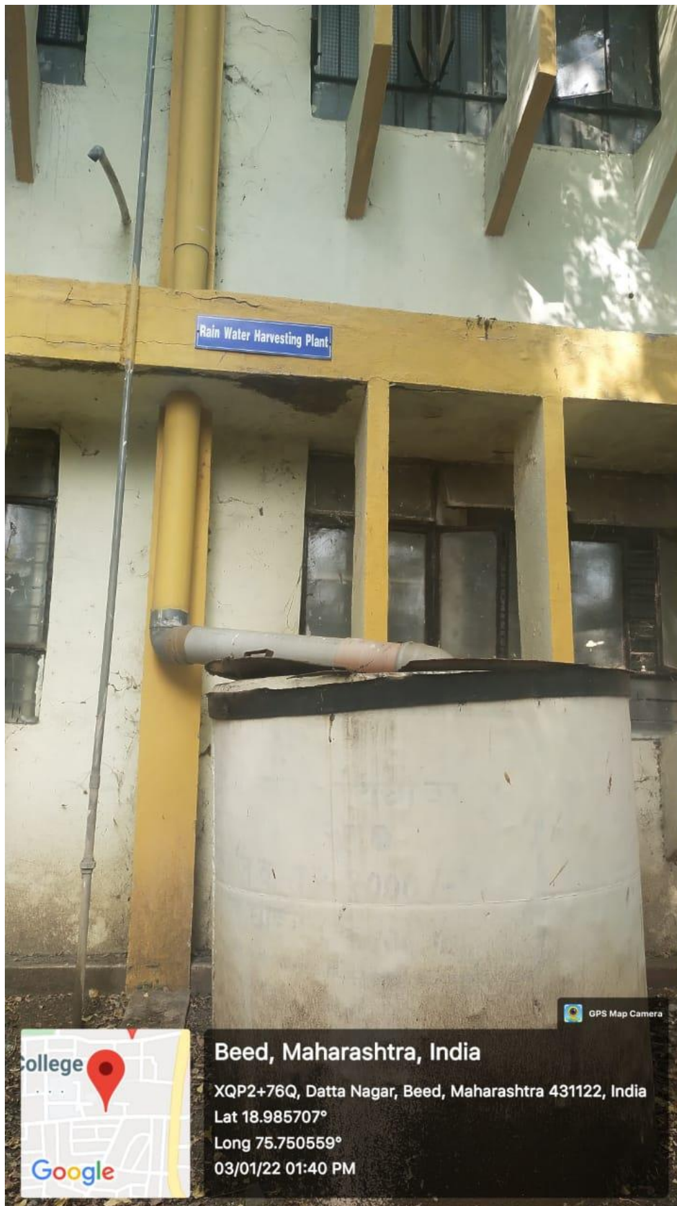
Bore well recharge plant
